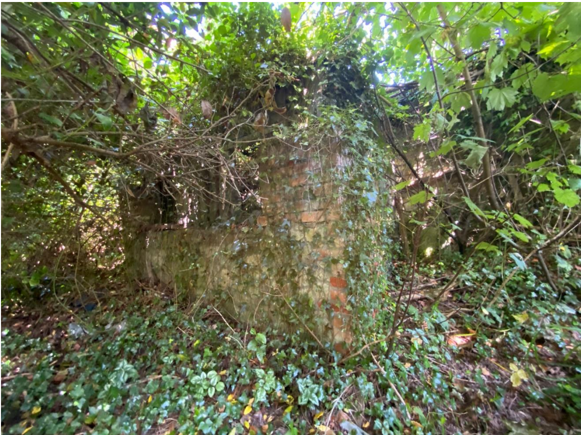
Plate 3. Old brick ruin located behind the small bungalow.
