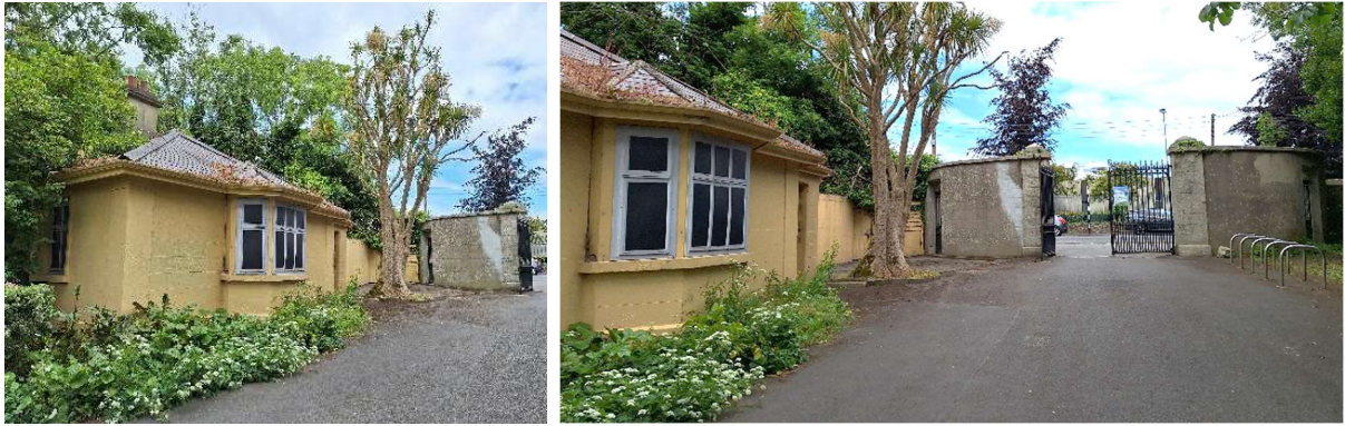
Fig. 14, 15 Front south-eastern elevation of gate lodge and entrance gateway.
