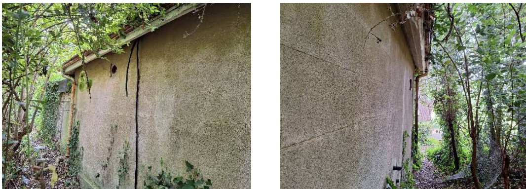
Fig. 22, 23 Rear north-western elevation with modern flat-roofed extension to north-east.
