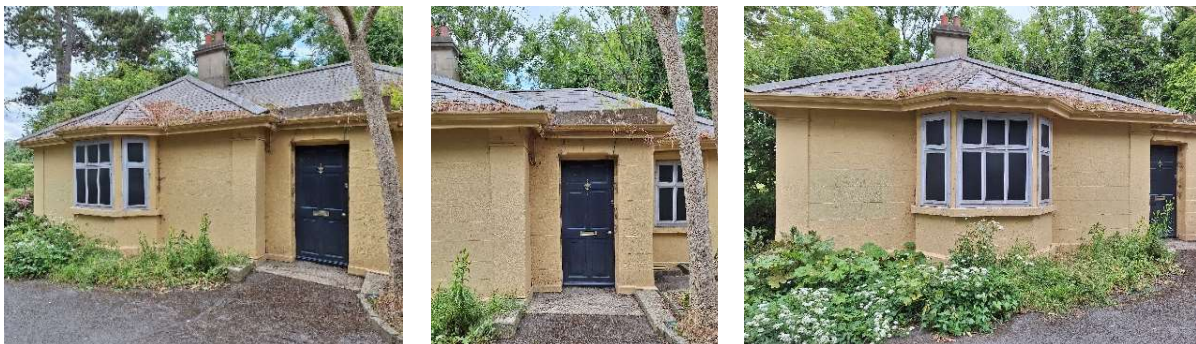
Fig. 8, 9 & 10 Projecting bay window and entrance to south-eastern elevation.
