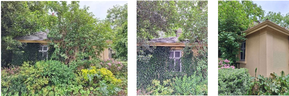
Fig. 17, 18, 19 Side south-western elevation with two square-headed windows and corner detail.
