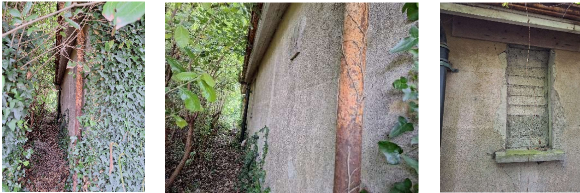
Fig. 20, 21 Rear north-western elevation with only one narrow ope.
