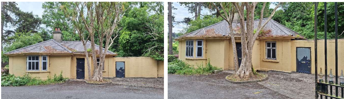
Fig. 6 & 7 Principal front south-eastern elevation.
