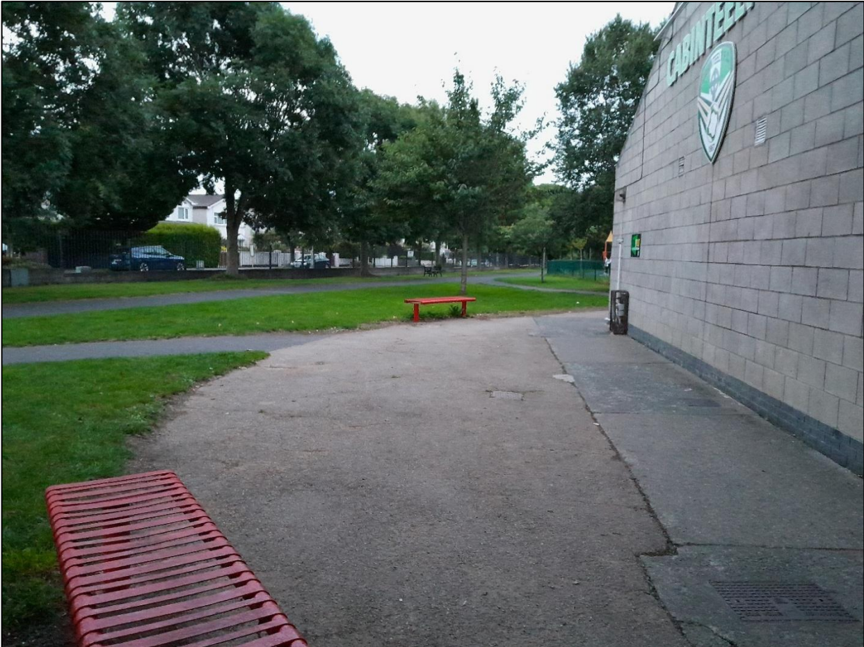
Figure 3-2: Main building and tarmacked paths running through the site
