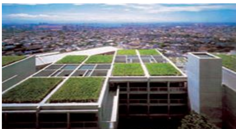
Examples of Extensive Green Roofs
