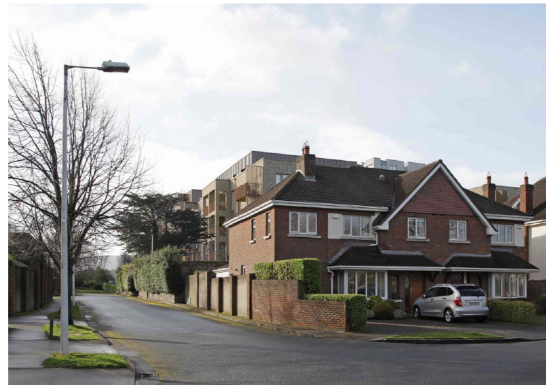
GRANTED SHD (CURRENTLY UNDER JURIDICAL APPEAL. PREPARED BY MODEL WORKS) - VIEW OF THE DEVELOPMENT FROM NORTH-EAST
