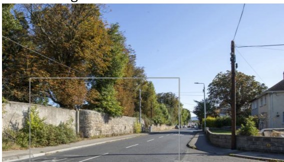
Fig. 8 Existing boundary wall
