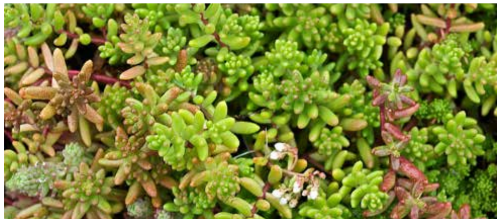
Green Roof/Sedum Roof
