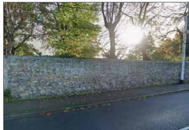
Existing Wall Retained
