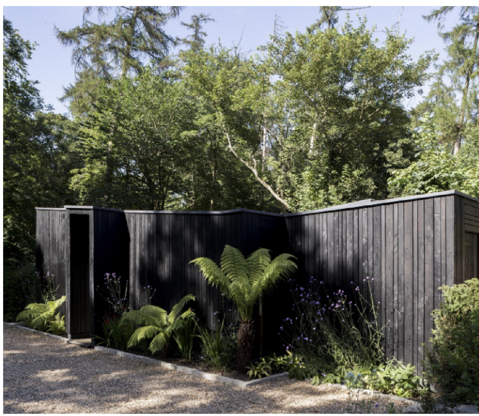
Visual Example of Bin and Bike Store Finish
