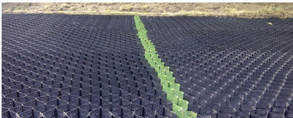
Image 10 - example cellular confinement system which may be implemented in bike shelter area.
