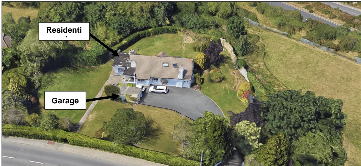
Figure 3.0 3D image of the dwelling and associated garage proposed for demolition.
