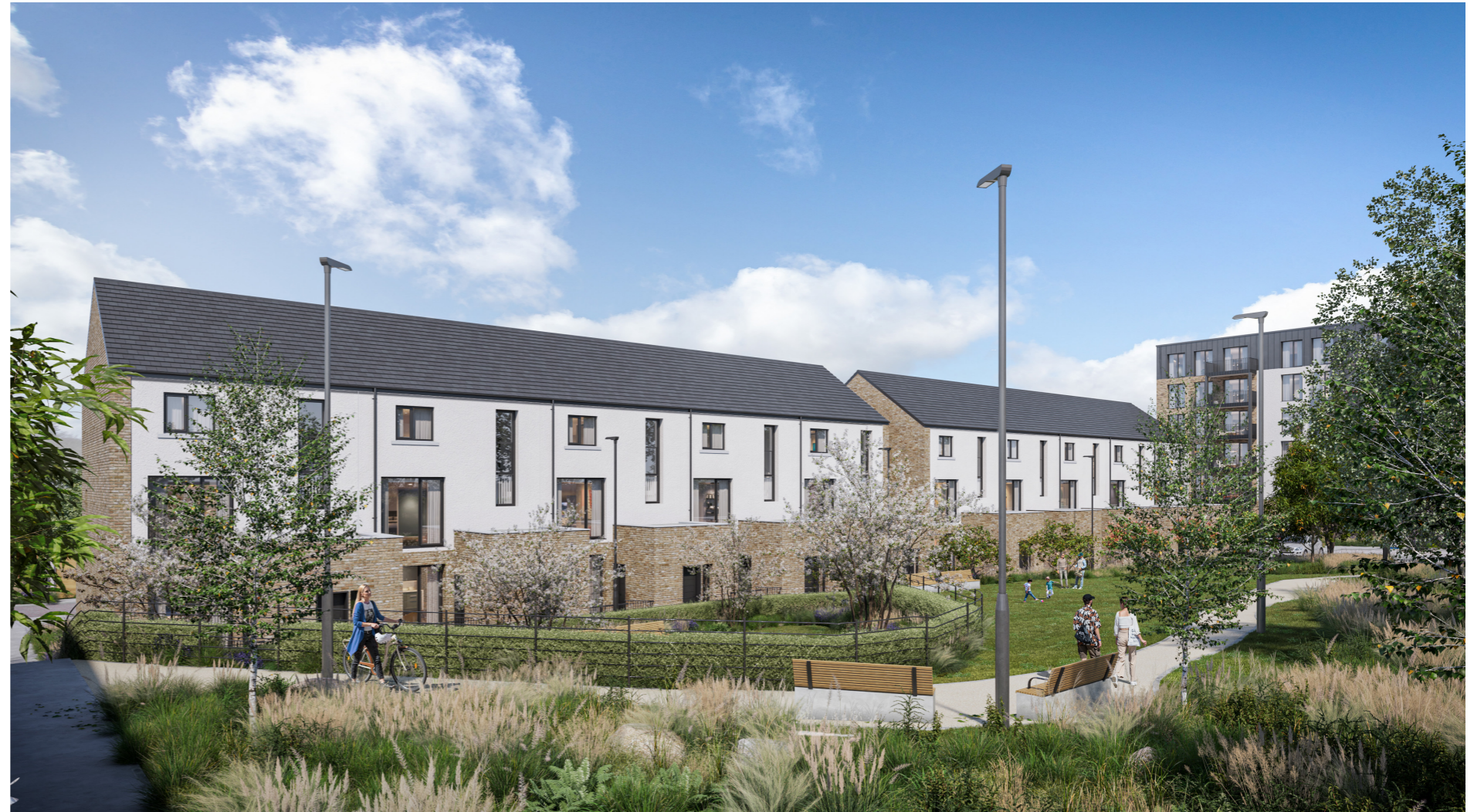
VIEW OF BLOCKS 1 & 2
