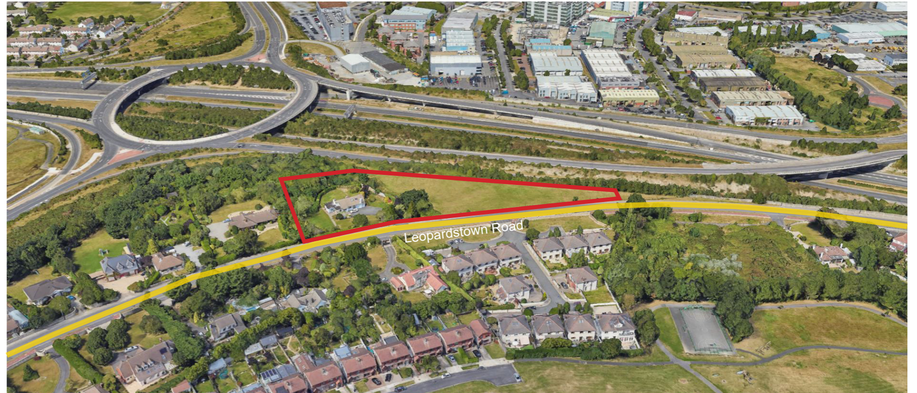
AERIAL VIEW OF SITE TO THE NORTH, WITH ADJOINING CONTEXT
