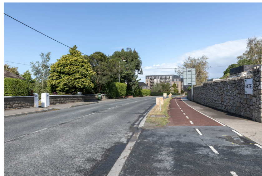
VIEW OF BLOCK 2 FROM WEST
