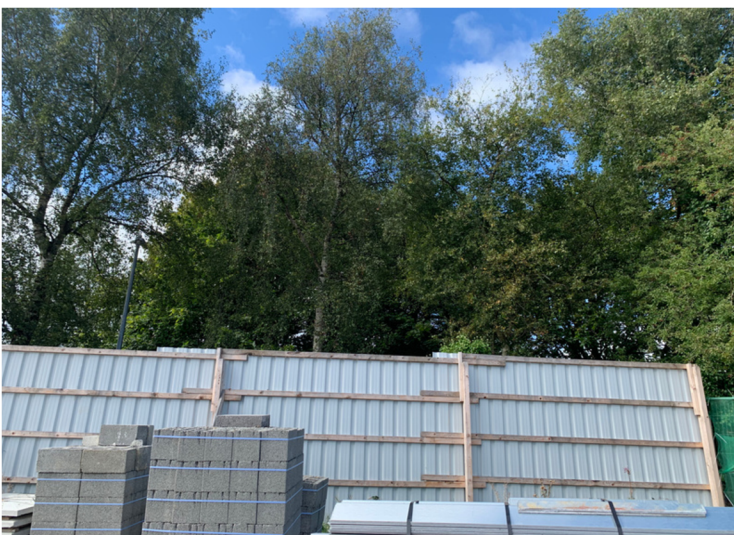
IMAGE 4: MATERIALS STORED OUTSIDE OF TREE PROTECTION FENCING
