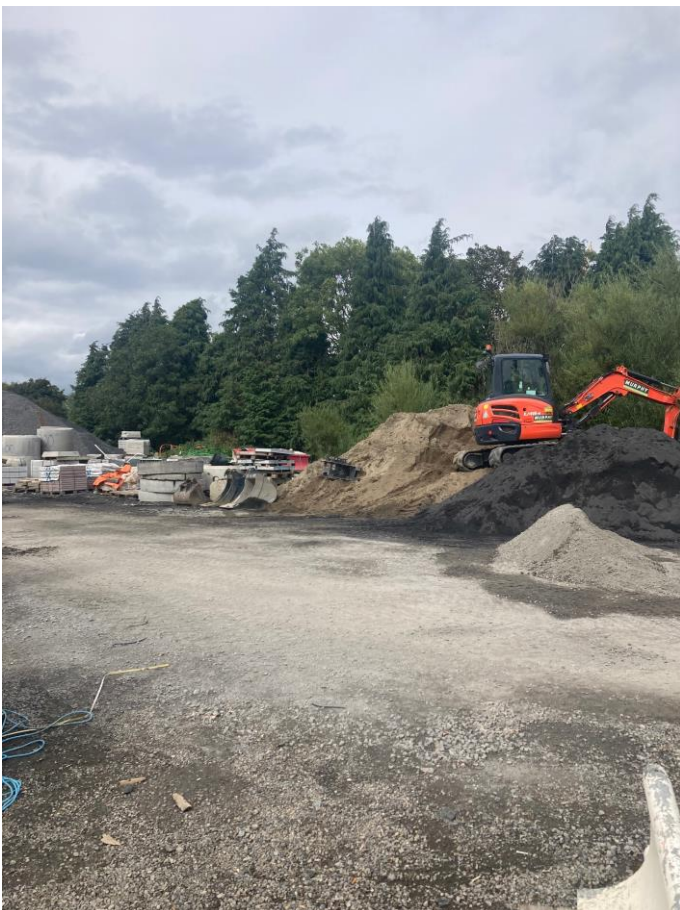
Image 4. View of Leyland cypress on northern boundary from existing site.
