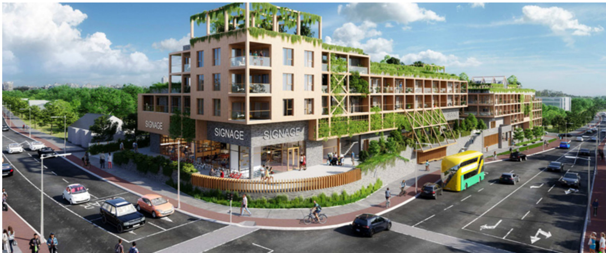
Image 19: Approved mixed use scheme Reg. Ref D23A/0456 on site opposite proposed development. Sandyford Road on right
