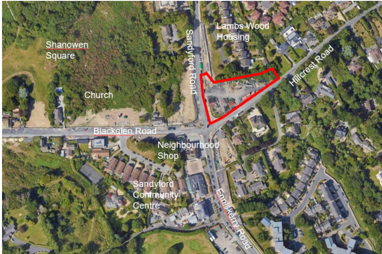
Image 2: Aerial view of the Lambs Cross Site c.2022- Evidence of its recent use as a site compound is visible
