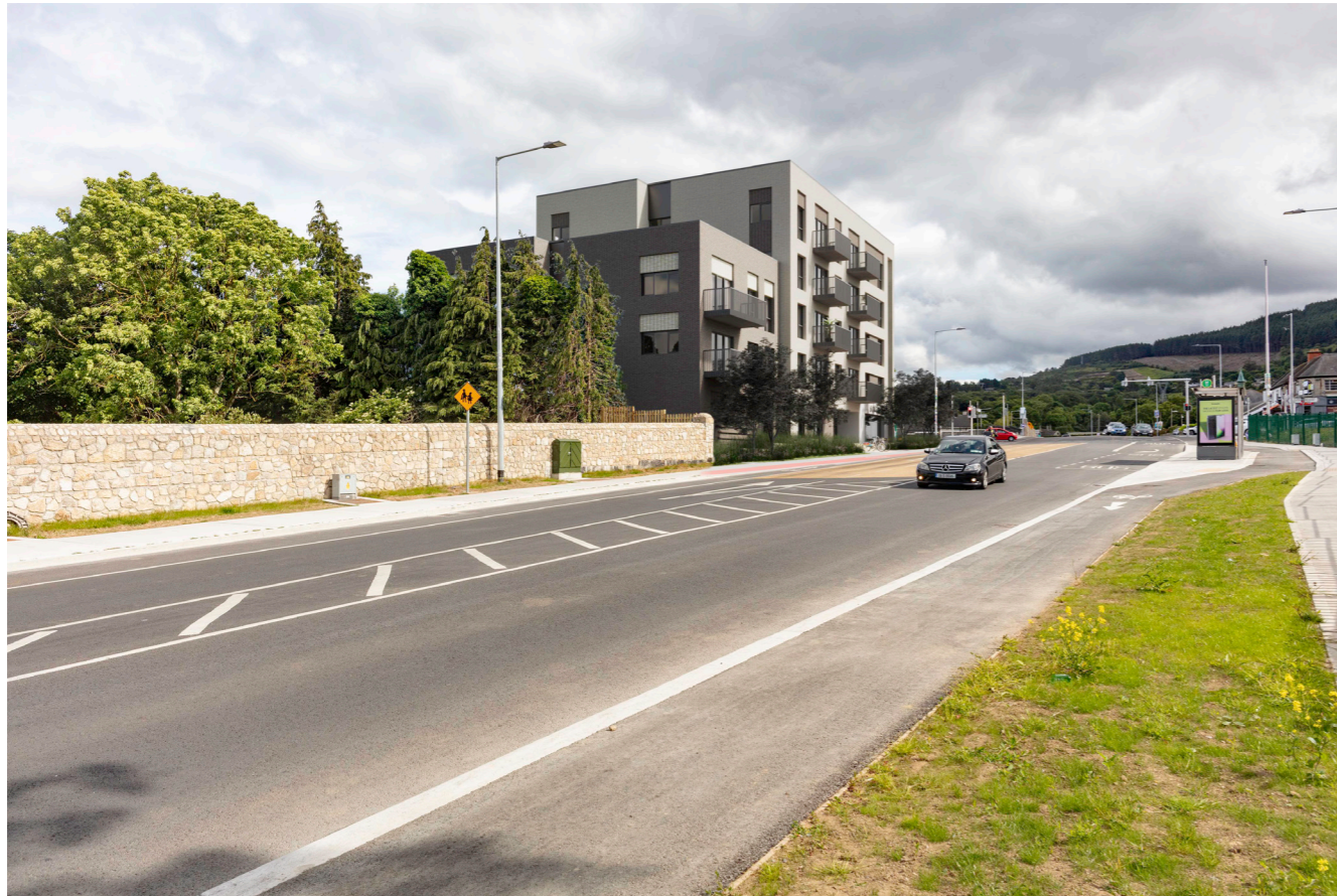
Image 35: View of proposed development from the northern approach along Sandyford Road. The height and massing of the block is in proportion to the increased width of the upgraded roads infrastructure at this location, forming part of a new neighbourhood hub
