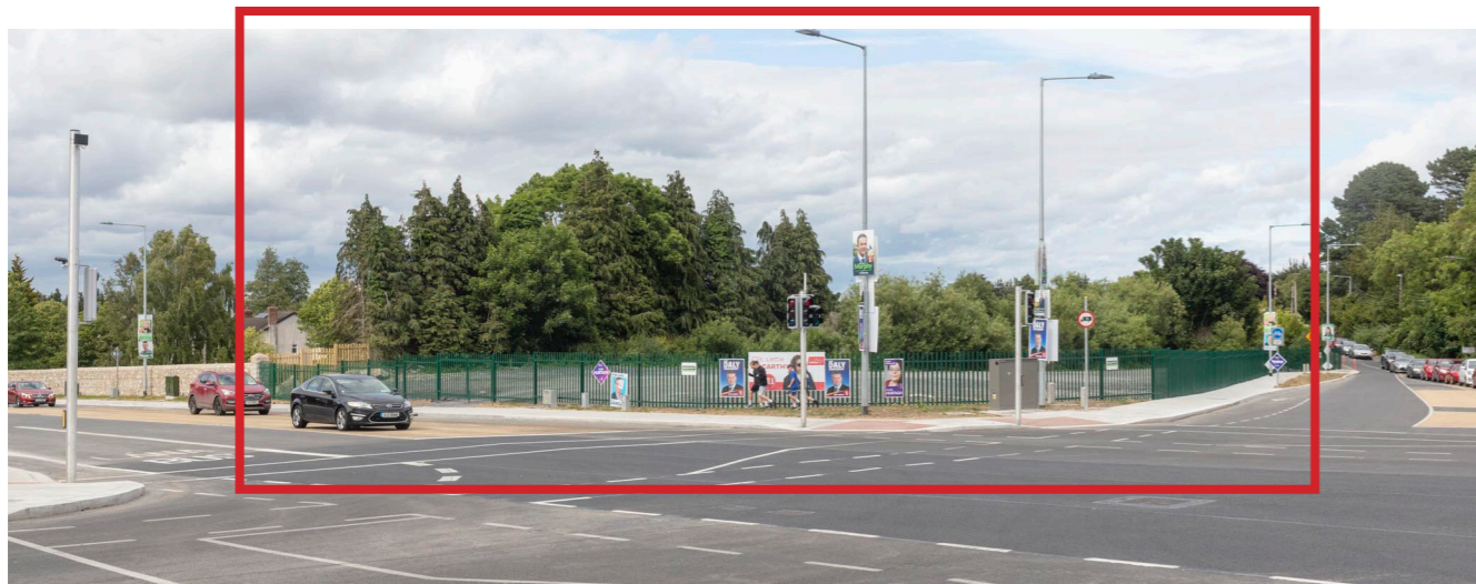
Image 3: Street View image of Site from the opposite corner of the intersection at Sandyford Road (June 2024) showing the recent road improvements and installation of fencing
