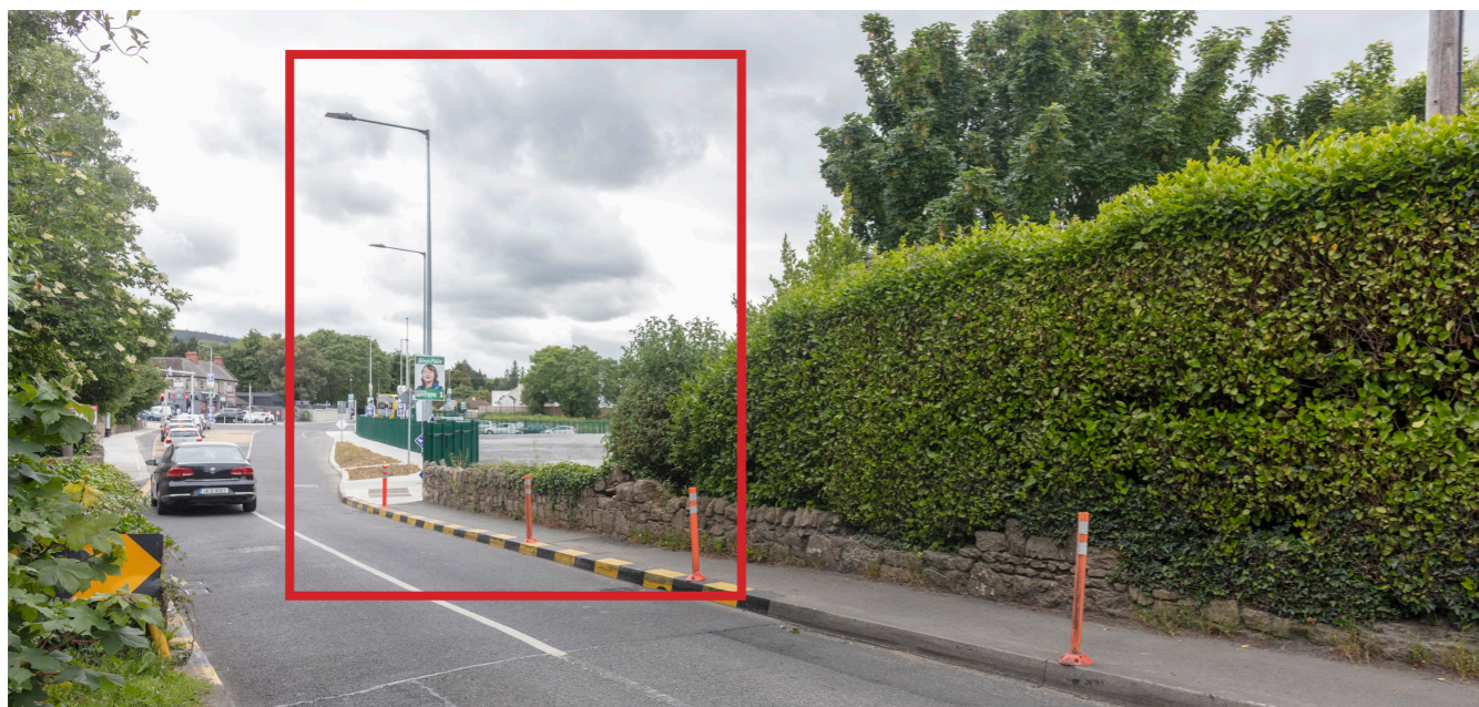
Image 9: Street View image of Site from the eastern approach (June 2024) along Hillcrest Road. The recent road widening works have been complete and narrows into the existing width of Hillcrest Road
