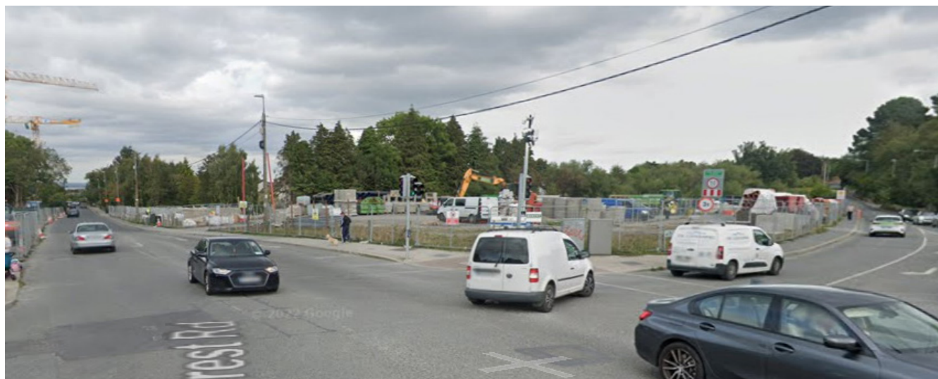
Image 13: 2022- Much of the vegetation removed. The site in use as a compound for the roadworks
