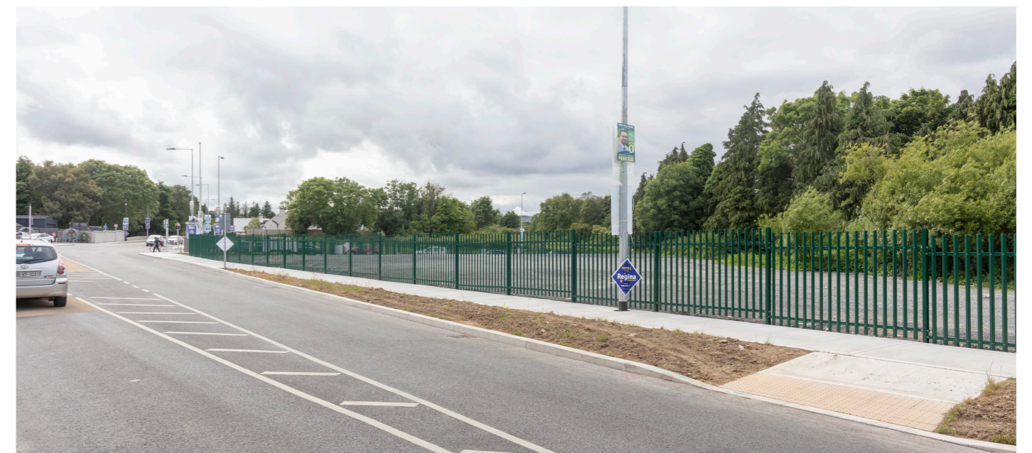
Image 10: Street View image of Site frontage (June 2024) to Hillcrest Road. The recent road widening works have been complete and narrows into the existing width of Hillcrest Road
