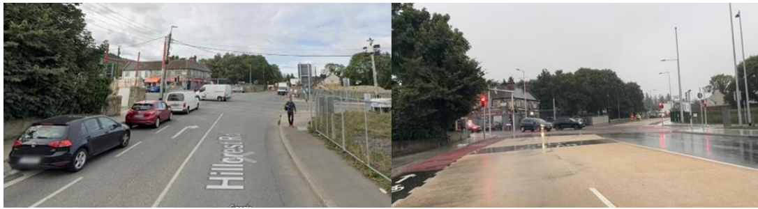
Figure 4-5 – Hillcrest Road Layout (Before on the left and After on the right)
