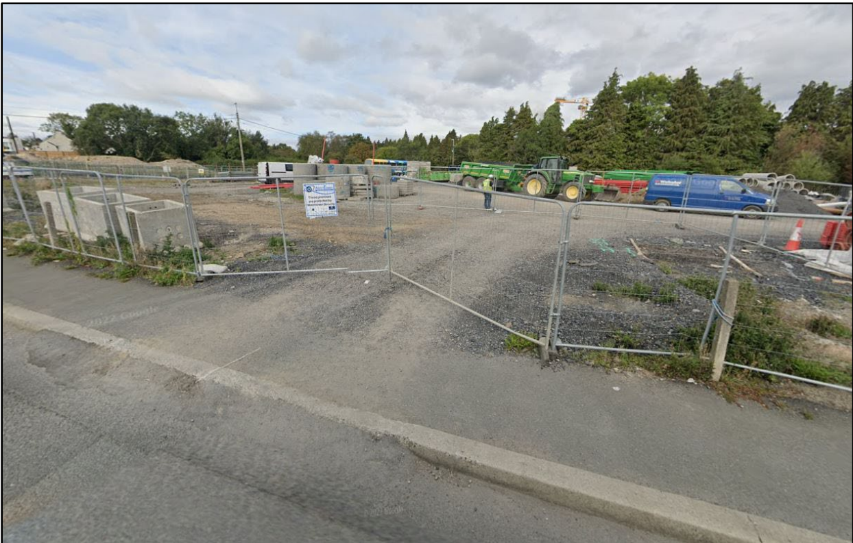
Figure 5.1: Site access point (Source: Google Maps).
