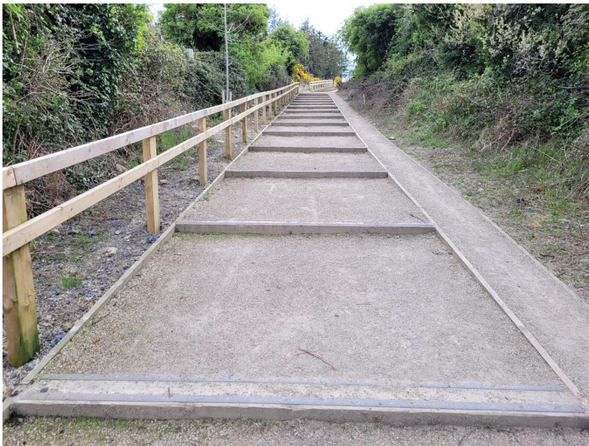
Figure 3.10.5: Example of Sloped Steps Used in Ticknick Park, Dublin
