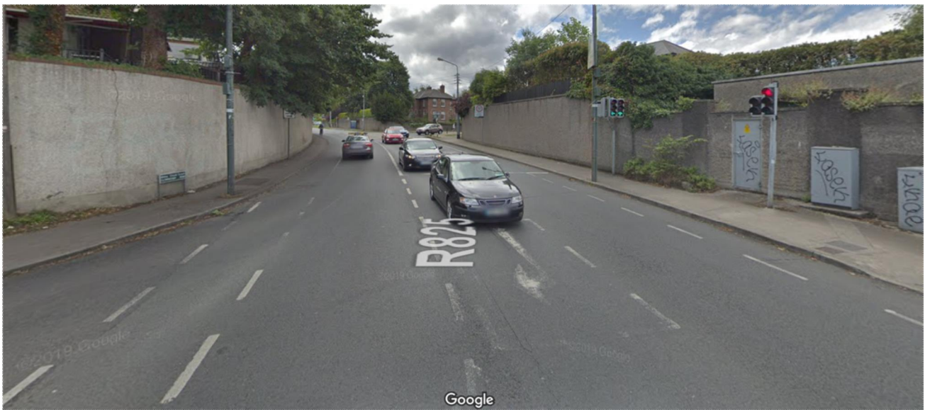
Figure 1: Extract from Google Streetview showing the location of the 'pinch point' and where the right turn onto Beech Hill Road will be removed
